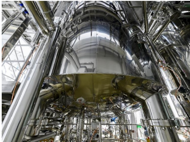
Bioreactor Kyowa Kirin Takasaki Plant (Gunma Prefecture)
