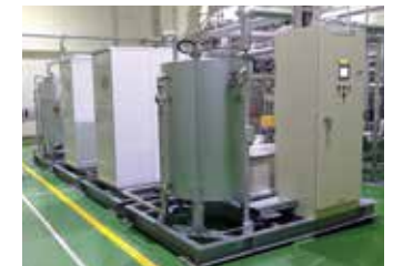
Heat pump at Shinshu Beverage
