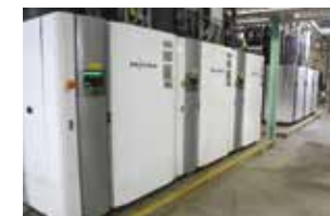
High-efficiency package boilers
