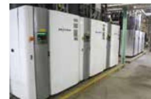
High-efficiency package boilers
