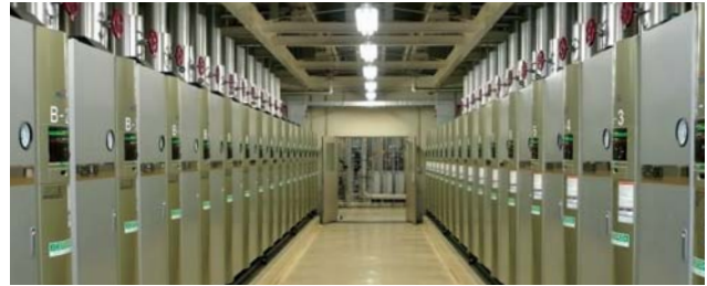
Rows of gas boilers
