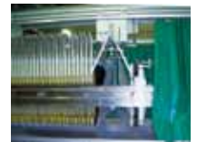
Phosphoric acid-recovery facility
