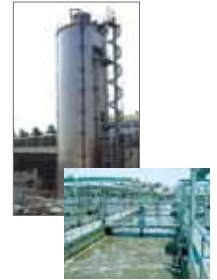
Wastewater-treatment facilities (Top: Anaerobic treatment facility; Bottom: Activated sludge treatment facility)
